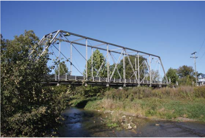
Linville Creek Bridge —Built in 1898 by the Wrought Iron Bridge Company of Canton, Ohio, the Linville Creek Bridge is Virginia’s only surviving example of a whipple metal truss bridge. This bridge is recognized on the National Register of Historic Places and the Virginia Landmarks Register.
