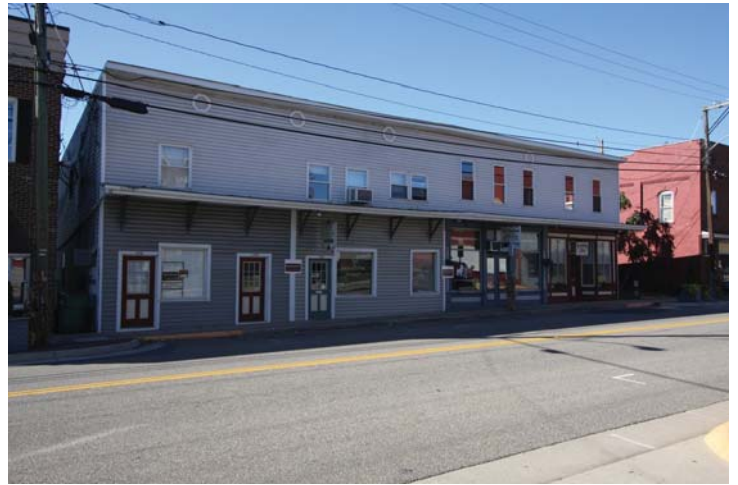
Broadway Motor Company —Located in the heart of the Broadway Business District, this nearly original commercial building dates back to the early 1900s. A Ford automotive dealership was housed here during the time of the Model A and Model T.
