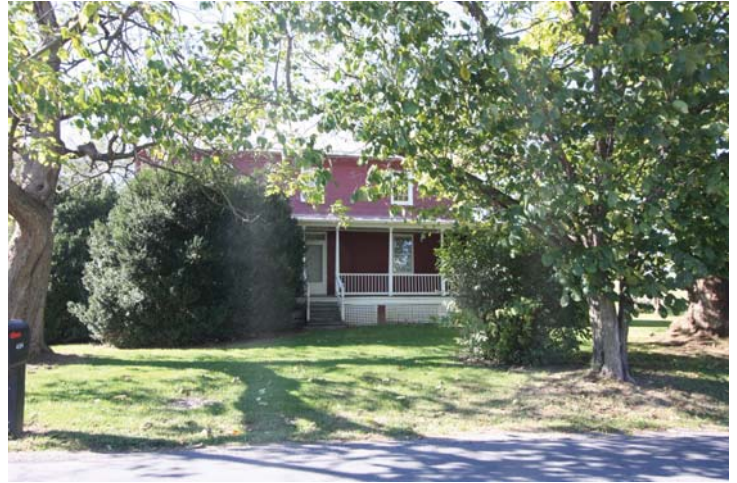
Elder Hays/Samuel Kline House —The home place of George Kline was built in the 1840s. The house is a subsequent one with three brick walls. It is I-shaped with several rooms and fireplaces. Much of the structure has been unaltered and all doors and windows are original.
