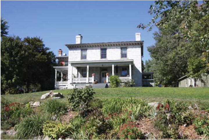
L.E. Hoover House —The L.E. Hoover House, built in the 1850s, is an interesting example of two, one-pile central hall plans which have been attached. It is the only antebellum stone building in the greater Broadway area.
