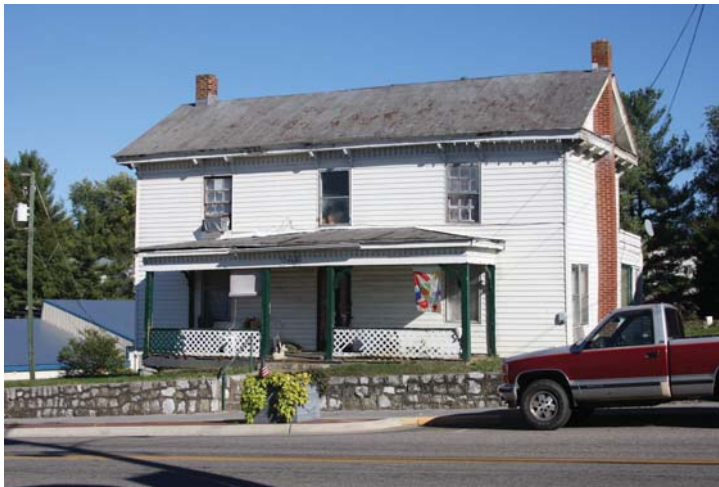
G.W. Baldwin House —A well preserved example of a decorated I-house that was built in the 1880s. The dentil cornices are typical for the area but the board and batten is not.
