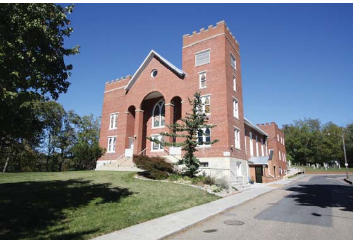
Broadway Presbyterian Church and Cemetery —Built in 1926, the Broadway Presbyterian Church is a well preserved example of churches constructed during this time. Much of the original interior is still in place and few changes have been made.
