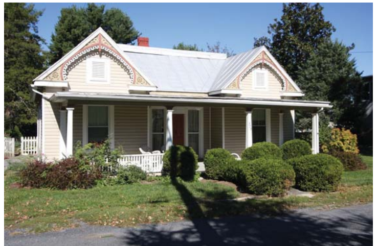
Montague House —Built in 1900, this Victorian style home is one of the most decorative homes found in Broadway with its cross gables, decorative bargeboards, cornice brackets and decorative glass doors.
