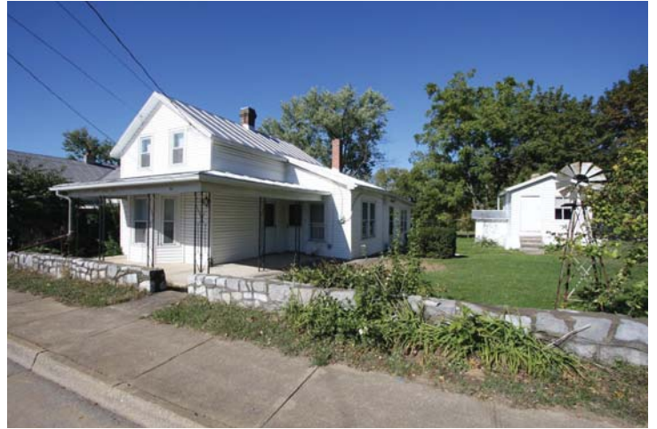
Leon Good/Workers House —One of four houses built for workers at the pottery factory during the boom time of the 1890s. This house is one of the two board and batten homes which was not common for homes built during that time.
