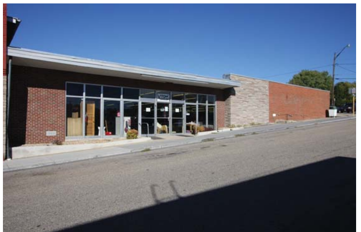
A.W. Whitmore, Store #2 —The A.W. Whitmore Store represents commercial architecture at the turn of the century. Renovations have occurred to give the first floor a more modern appearance.
